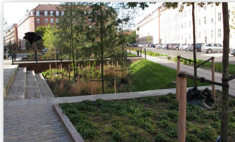
Storm water storage space at Tåsingeplads in Copenhagen, Denmark
